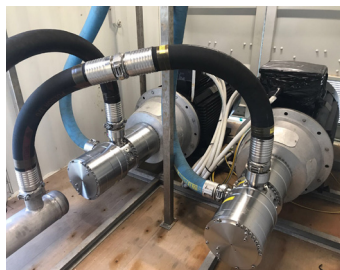
iSave 70 energy recovery devices, APP 86 pumps, VLT® AQUA Drives, and DST P401 pressure transmitters in the Sarlux SWRO plant
