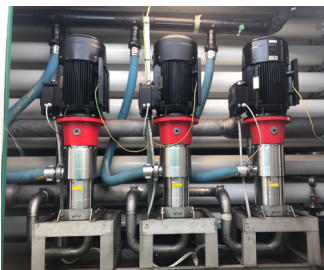
iSave 70 energy recovery devices, APP 86 pumps, VLT® AQUA Drives, and DST P401 pressure transmitters in the Sarlux SWRO plant
