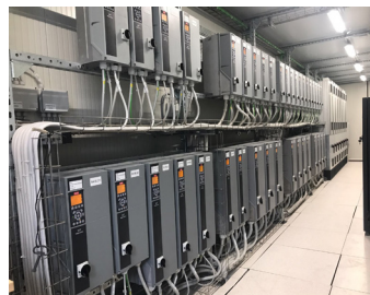
iSave 70 energy recovery devices, APP 86 pumps, VLT® AQUA Drives, and DST P401 pressure transmitters in the Sarlux SWRO plant
