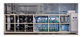
Danfoss offers a range of pack controllers for use in compact systems, as well as in large power packs. The ADAP-KOOL® pack controllers ensure efficient control and operational reliability for advanced solutions for controlling up to twelve compressors. The intelligent controllers optimize the suction and condensing pressure according to load and outdoor temperatures.
