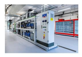
In the Danfoss Smart Store the cooling and heating technologies are in operation 24/7 and run exclusively on natural refrigerants ( $CO_2$ ). It's not a laboratory simulating real-life operation. Customers open cabinet doors hundreds of times a day and every time it puts demand on the cooling and heating of the supermarket. The Danfoss Smart Store demonstrates our available solutions in action.
