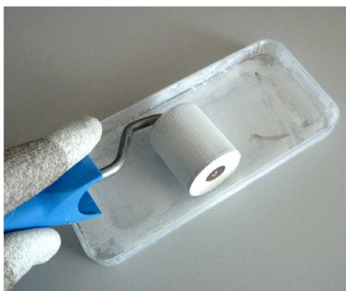
Figure 6: Working the paste onto the roller using a hard plastic tray
