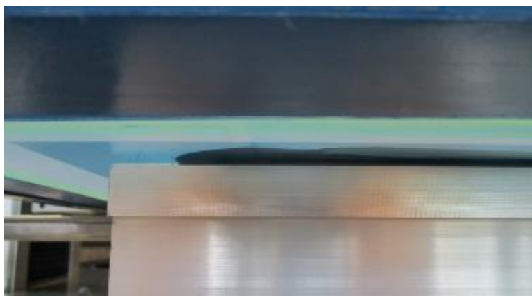
Figure 11: Underside of screen showing gap
