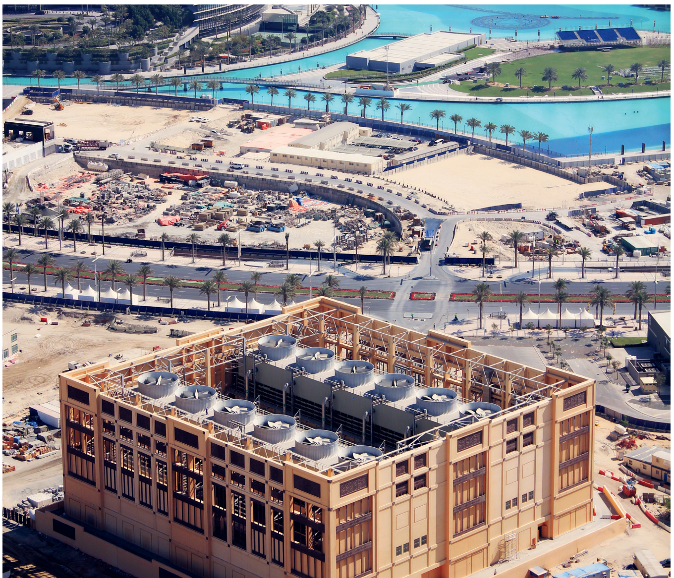
Figure 9. District cooling plant using wet cooling towers.
