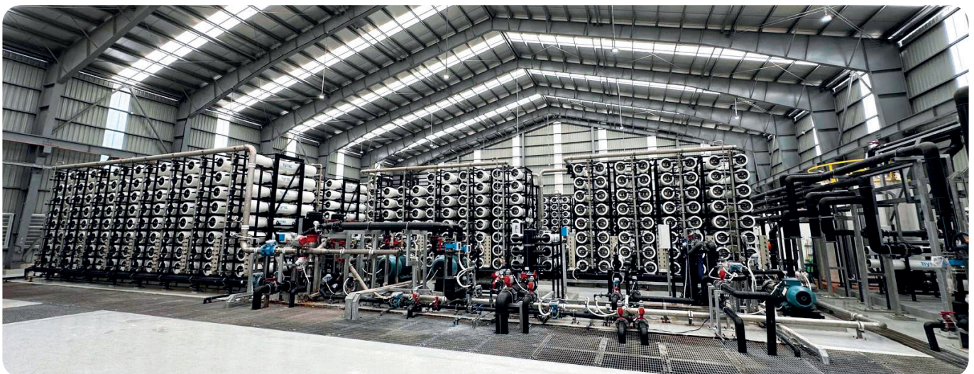
Whole Hyrec plant consisting of both SWRO and OARO trains.
