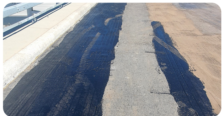
Fig. 1. DEVlasphalt™ heating cable under the first layer of Road asphalt rolled by a hand drum
