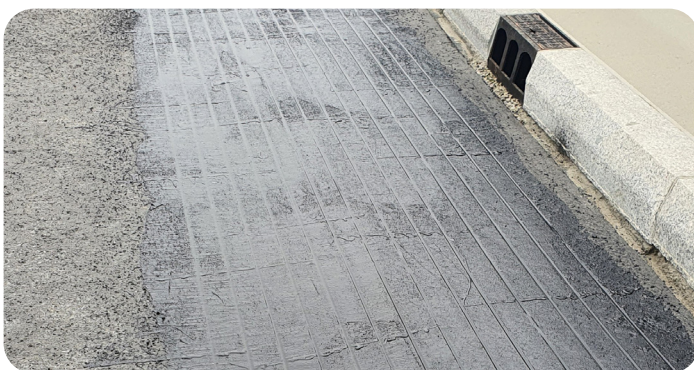
Fig. 1. DEVlasphalt™ heating cable under the first layer of Road asphalt rolled by a hand drum
