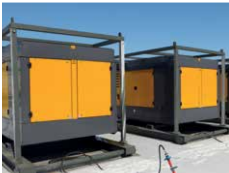
Variable speed technology helps reduce the size of power backup systems.
