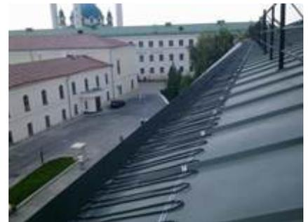
5. The selected cable should work as integrated part of an installation in the gutter and drain pipe, so connect it to the same control, e.g. ECtemp 850.
