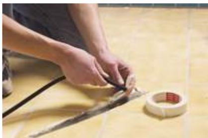
4. Install conduit pipe for floor sensor (must be sealed at the end). Check resistance of sensor before installing in pipe. Install wire sensor in pipe.
