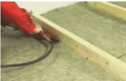
4. Apply mesh or foil onto the insulation. Fasten it to the joists.
