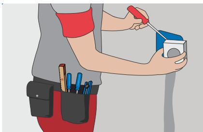
7. Check the insulation resistance and resistance (Ohm) rating of the heating cables. Plaster the wall groove and connect the cold tail, sensor and thermostat. Check resistance of sensor.
