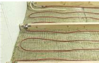
7. Install the heating cable evenly over the whole floor area.
