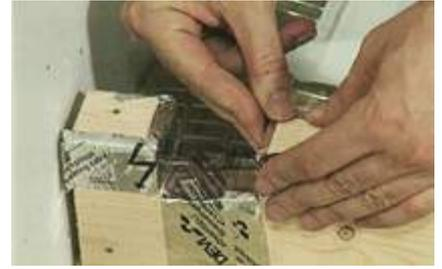
3. Recess has to be covered with metal or aluminum tape etc.
