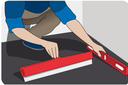
1. Make sure that the sub floor is reasonably level, firm and stable. New concrete needs to dry out for 30 days before installation.
