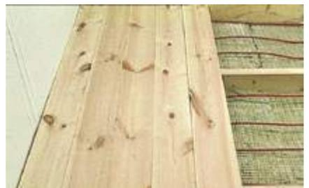
9. Install wooden surface. Check resistance and insulation value of cable and resistance of sensor and connect the thermostat.
