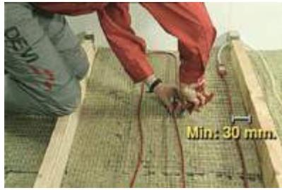
5. Install cable with chosen C-C distance. Max. 80 W/m<sup>2</sup> and cable output max. 10 W/m. Min. 3 cm distance to wood.
