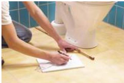
2. Check/draw a plan in order to position heated area, mat, cold tail, floor sensor, thermostat and connection box, if any.
