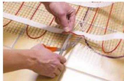
6. Cut and turn the mat mesh when meeting walls or obstacles. DO NOT CUT the cable.
