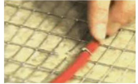
6. Fasten cable at max 30 cm intervals. E.g. plastic cable ties can be used. Secure that the heating cable does not rest in insulation.
