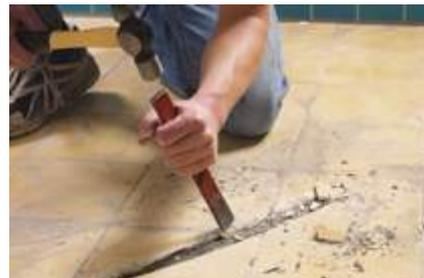
3. Make a groove for the sensor conduit pipe and cold cable.
