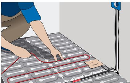
6. Check the insulation resistance and resistance (Ohm) rating of the heating cable before installation. Install the ECflex heating cable. Make sure that the cable end and connection muffs are in contact with the aluminum plate or aluminum tape at all times.
