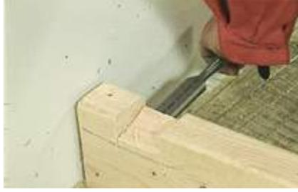
2. Cut 3x6 cm recess in joists. Check C-C to do minimum number of recess (best on one side / end of joists).
