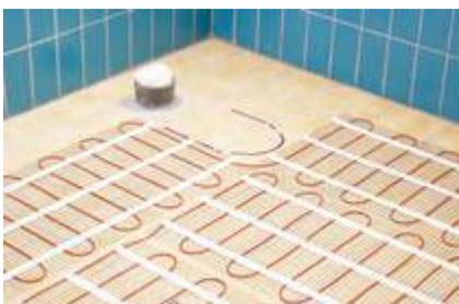
8. Install mat on the entire surface. App. 3-4 cm between nearby mats. Check resistance and insulation values of mat and resistance of sensor.
