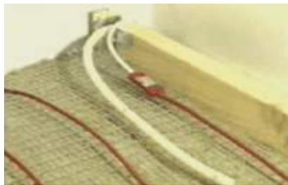
8. Install sensor pipe and wire sensor. Seal/close the end of pipe. Check resistance and insulation value of cable and sensor's resistance.
