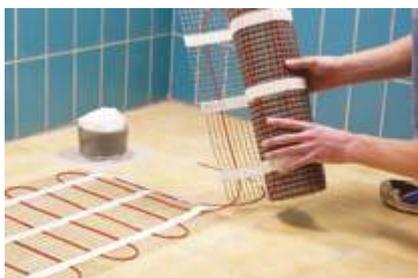
7. Install the heating mat avoiding obstacles, future objects fixed to the floor, etc. Min. 3 cm between any two cable lines.
