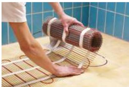
5. Check resistance and insulation values of the mat. Roll out the heating mat from thermostat position. Attach it to the sub floor.
