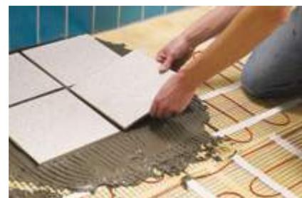
9. Apply tile glue and Install tiles. Check resistance and insulation values of mat and resistance of sensor.
