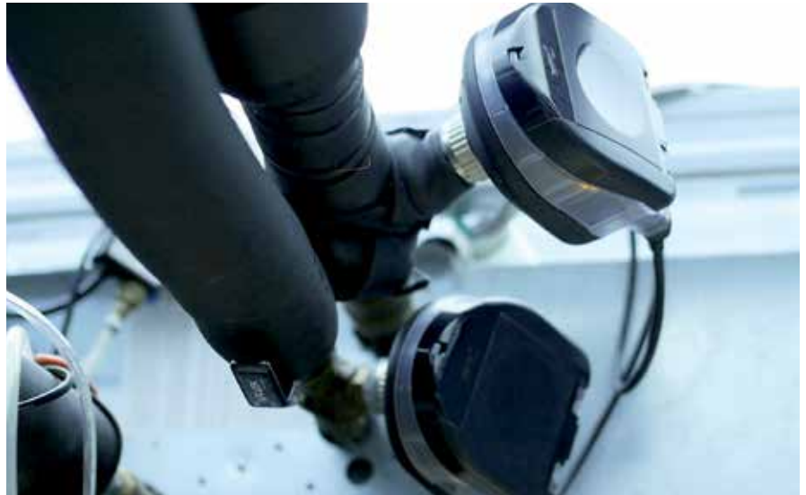
NovoCon® actuator in combination with AB-QM valve
