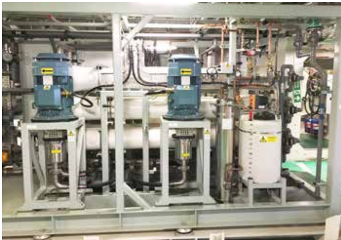
RO desalination plant with two APP 8.2 pumps in parallel
